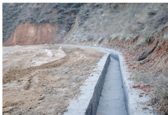
矸石场坡顶一侧排水沟
